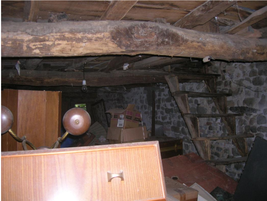
Piano terra Cantina
